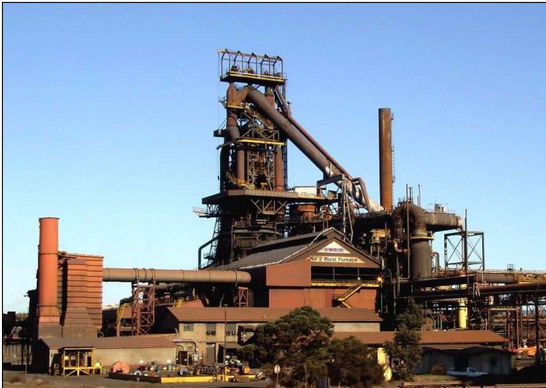
Whyalla Blast Furnace
