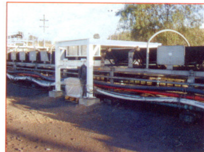
Side view of typical Coalscan 1500 installation, showing the detector below the conveyor belt and the electronics cabinet on the ground before being installed on side mounting.
