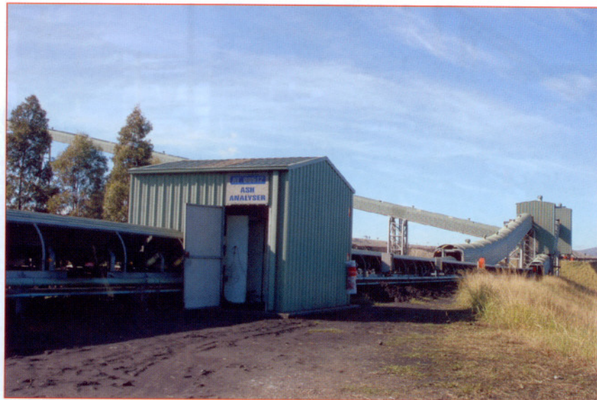
Shed in which Coalscan 3500 is installed.
