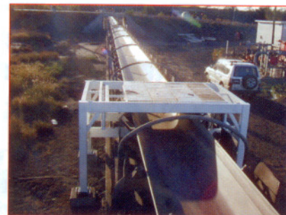
Top view of typical Coalscan 1500 installation, showing lead shielding surrounding analysed coal.
